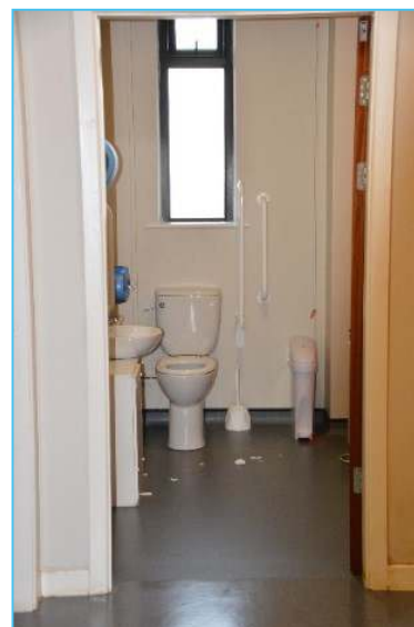
Figure 21. Lack of visual contrast in accessible toilets
