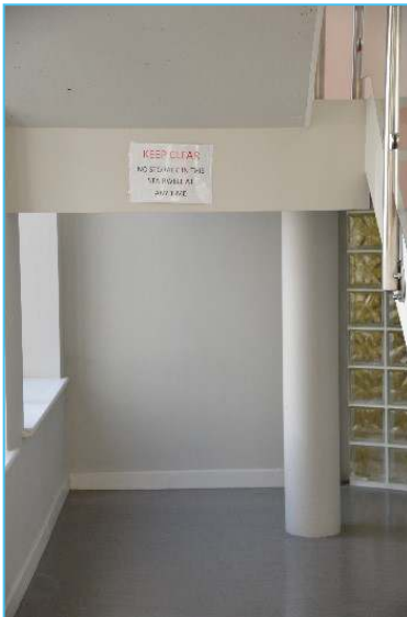
Figure 14. Low soffit under stairs ground floor
