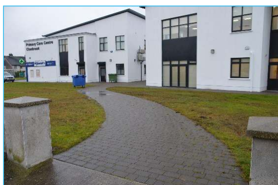
Figure 3. Standing water, and weeds.
