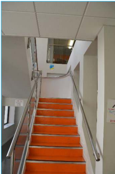
Figure 16. Stairs reflection in glass guarding and open-ended handrails.
