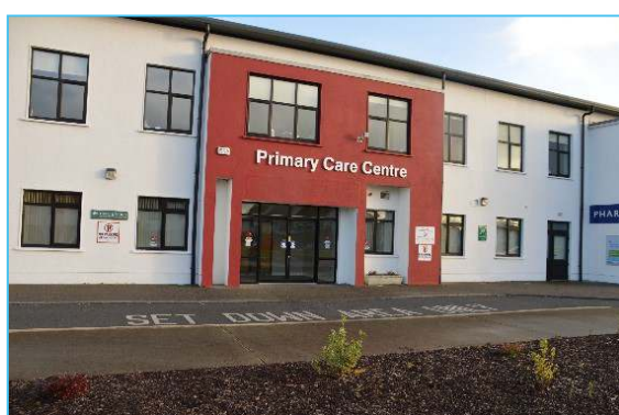
Figure 7. Main entrance is prominent on the west elevation. If doors contrasted with surrounding fenestration it would improve visual access.
