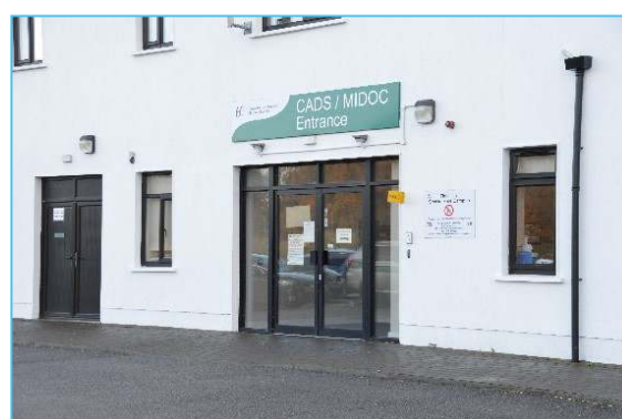
Figure 8. CADS and MIDOC entrance at rear of building. If doors contrasted with surrounding fenestration it would improve visual access.
