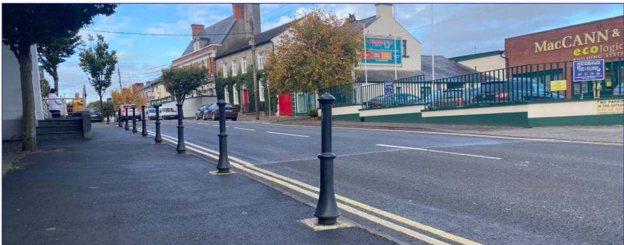
Bollards installed as part of upgrade work to address traffic management issues and prevent parking on footpaths.
